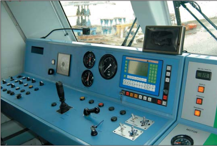
Driver's desk. Driving controls are on the left; fire-fighting functions are on the right.
